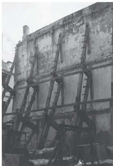
Timber raking shore
