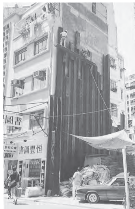
Steel sheet piling for basement excavation
