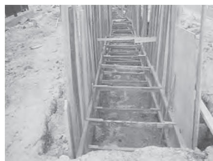
Timber planking and strutting for trench excavation
