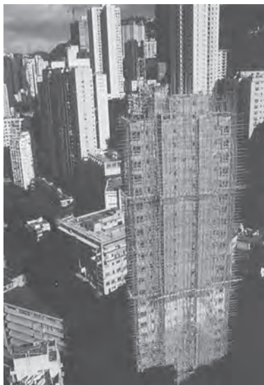
Residential tower at Bonham Road
