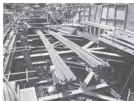
Steel strutting for basement excavation
