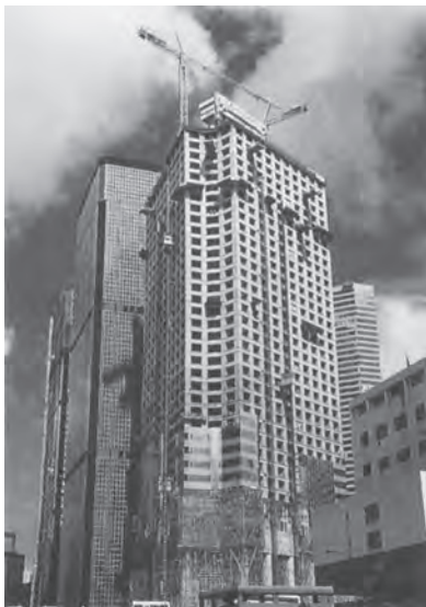
Central Plaza, the tallest office building located at the Wanchai waterfront, under construction
