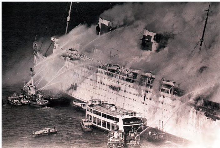
Figure 8.26. Burning Seawise University heeling over from the weight of water pumped on board (Ian Shiffman).
