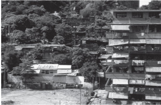
Figure 1.2: Mark II resettlement housing, Kwun Tong, 1982. Copyright and provided by Alan Smart.
