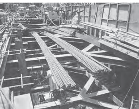
Steel strutting for basement excavation
