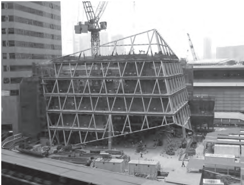
The construction of a diagrid structural frame
