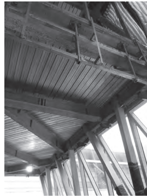
Construction of a composite metal deck
