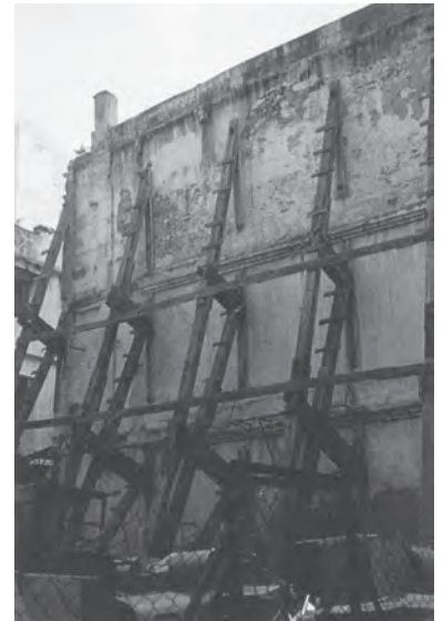
Timber raking shore
