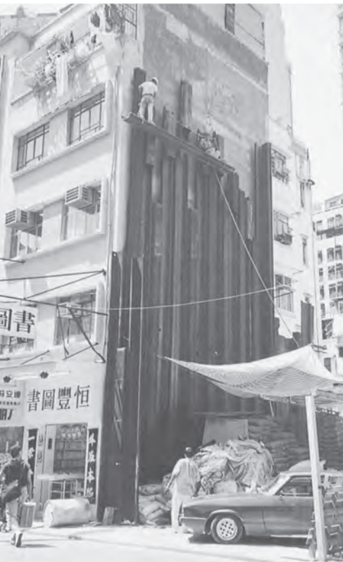
Steel sheet piling for basement excavation
