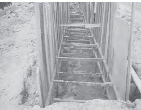
Timber planking and strutting for trench excavation
