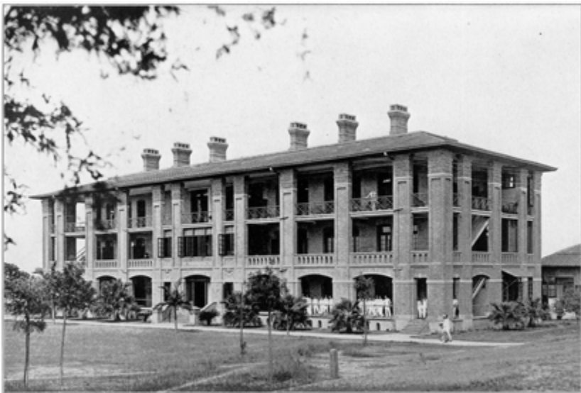
MARTIN HALL FROM THE SOUTHEAST. Named in memory of Mr. Henry Martin, of Cincinnati and Philadelphia. This building, 33 x 166 feet, was the first permanent one to be erected at the College, 1905-7, and also one of the first buildings with brick walls and reinforced concrete floors to be built in China. It is at present the only building for classrooms and laboratories for both the Secondary School and the College of Arts and Sciences. The entire north verandah is glassed in as a laboratory with every square foot in use, indicating the pressing need for a Science Hall with laboratories.
