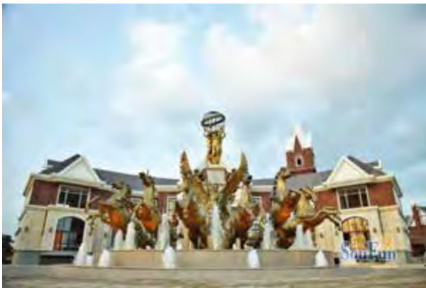
Fountains line the entrance to the English County development in Kunshan, which boasts to potential residents that its homes incorporate “classical English architectural concepts.” Photograph from SouFun.com.
